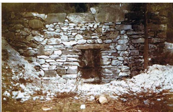
Lime Kiln – 1976 (after reconstruction)
